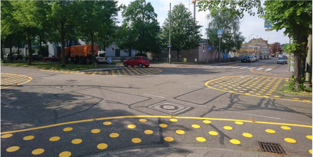
Figure 3 More space for pedestrians: curb extensions with polka dots
